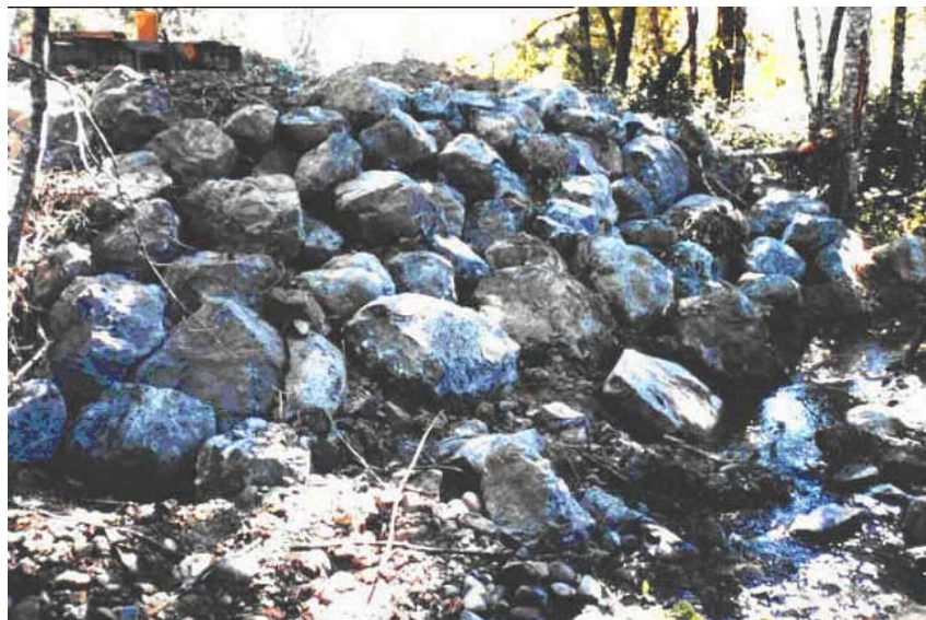
Figure 4 Riprap in place
