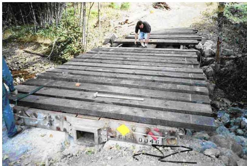
Figure 6 Putting on the new pressure treated planking
