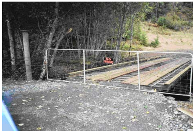
Figure 2 Post-project, Buck Fork Creek Bridge installed
