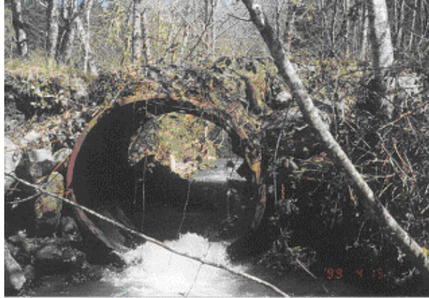
Figure 1 Pre-project view, Buck Fork Creek Culvert, outlet end
