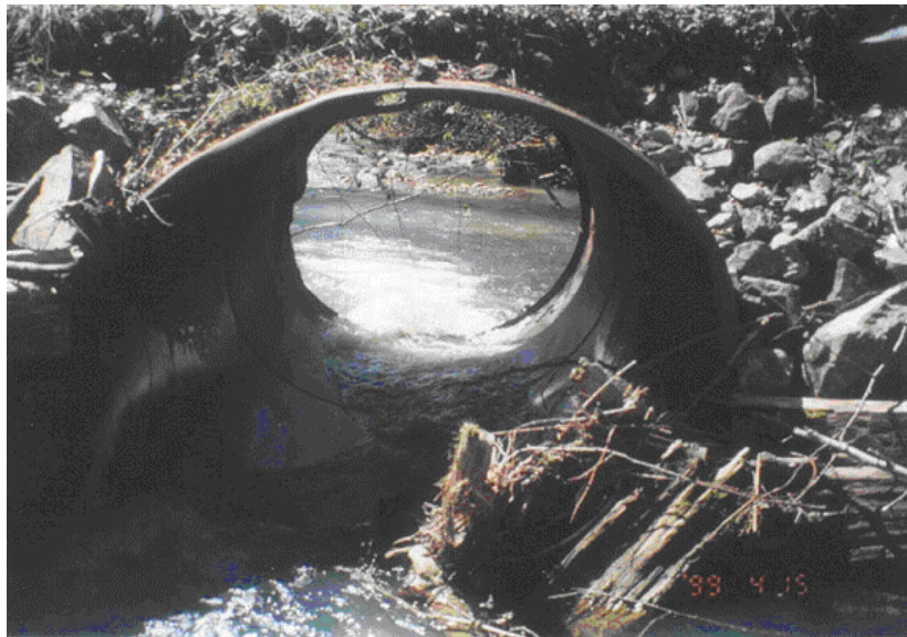
Figure 3 Pre-project, interior view of the old culvert
